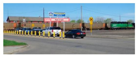
Figure 3. Non-traversable median at train crossing
