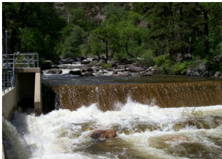
The diversion dam at our Intake Facility in Big Goose Canyon.
