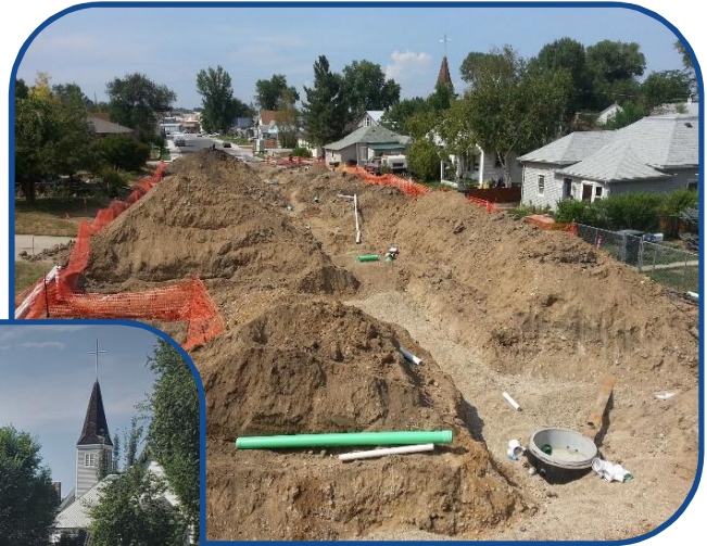
Wyoming Avenue – During Construction
