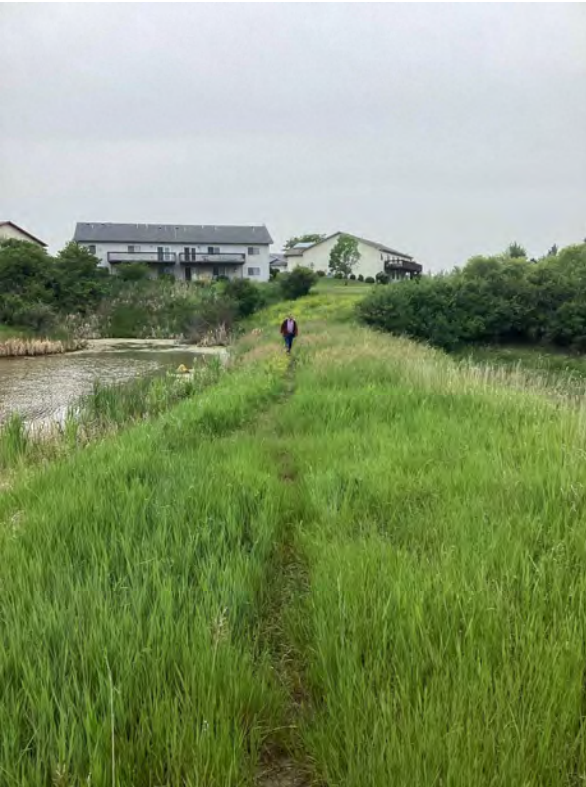
5.3 Holly Ponds No. 3 Reservoir - View of Dam (Looking Northwest)
