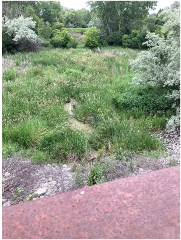
7.2 Holly Ponds No. 1 Reservoir - Outlet (Looking East)
