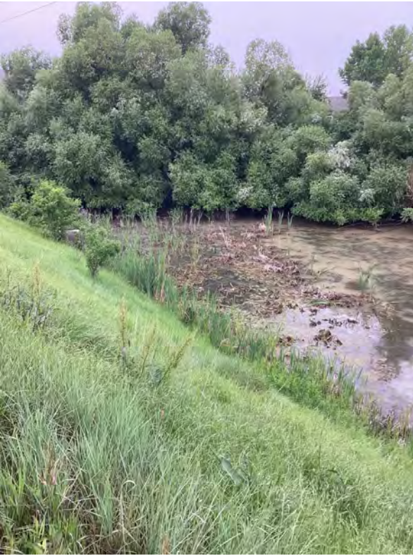
2.1 Holly No. 1 Reservoir - South End of Reservoir (Looking West)
