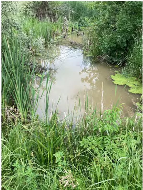
11.2 Mavrakis Pond - Inlet Culvert (Looking West)
