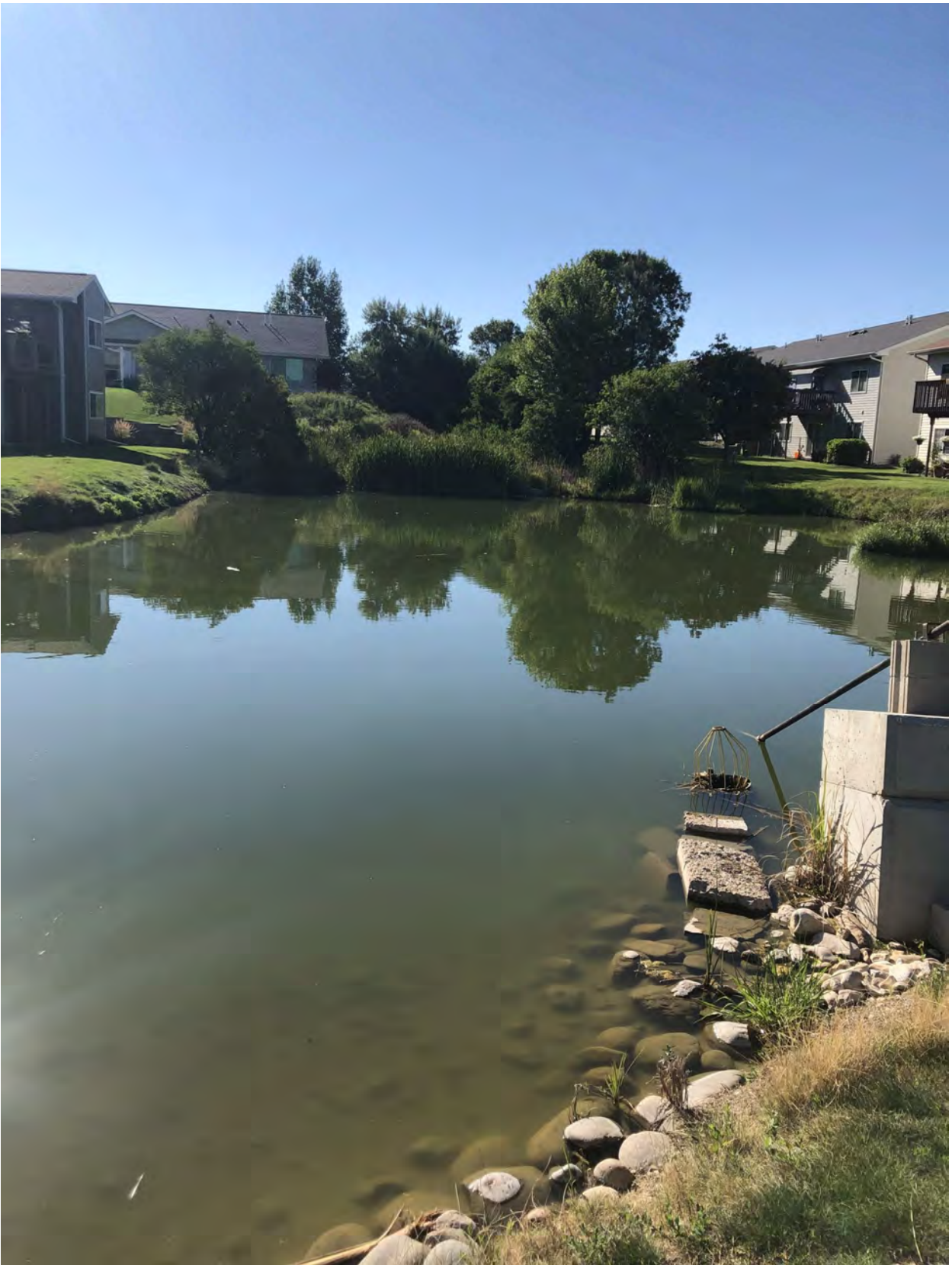
3.1 Holly No. 5 Reservoir - South End of Reservoir (Looking West)
