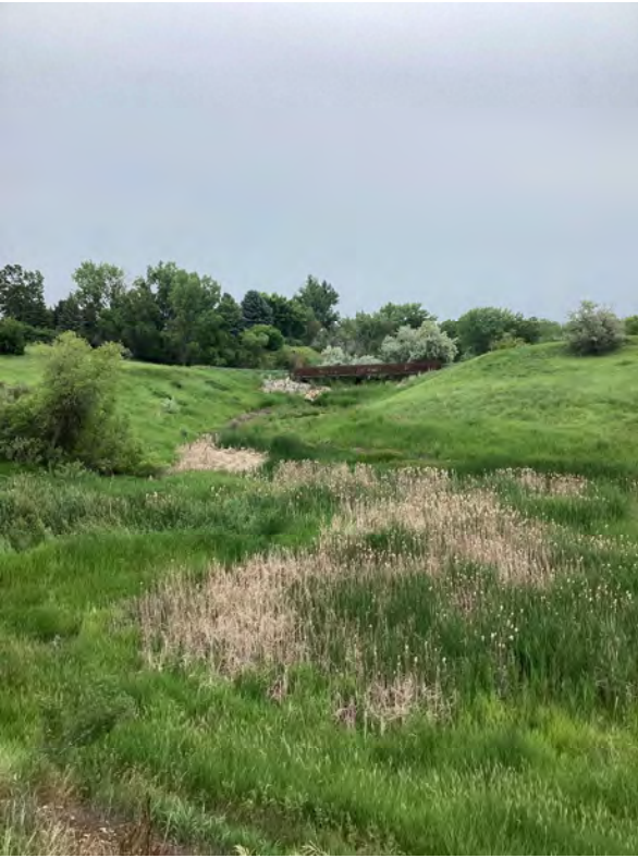
7.1 Holly Ponds No. 1 Reservoir - Reservoir Channel (Looking East)
