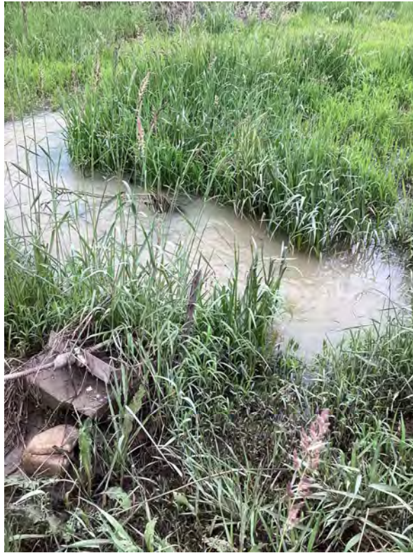
7.3 Holly Ponds No. 1 Reservoir - Gate Valve (Looking Southwest)
