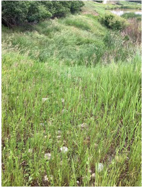
5.2 Holly Ponds No. 3 Reservoir - Emergency Spillway (Looking Northeast)
