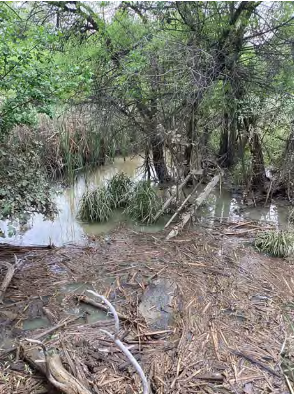
8.3 Holly No. 2 Reservoir - Gate Valve (Looking Southwest)
