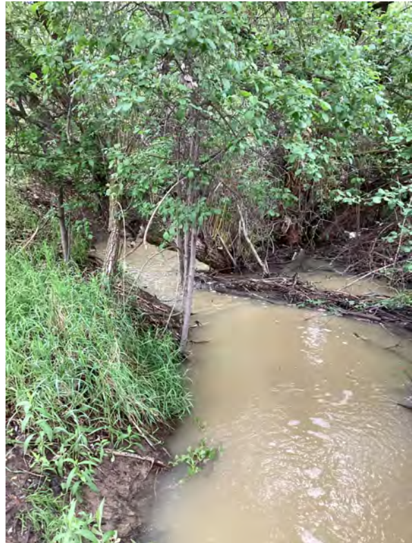
9.4 Hume No. 1 Reservoir - Emergency Spillway (Looking East)
