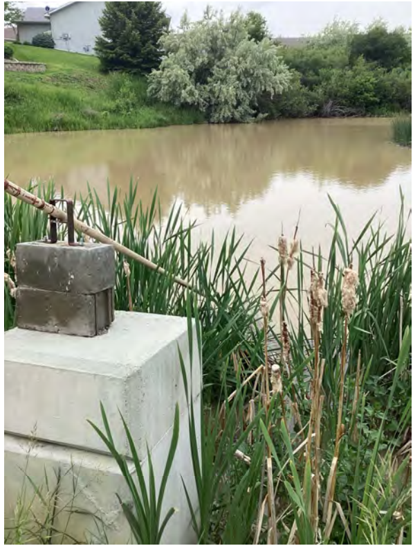
4.2 Holly Ponds No. 4 Reservoir - Outlet Structure (Looking West)
