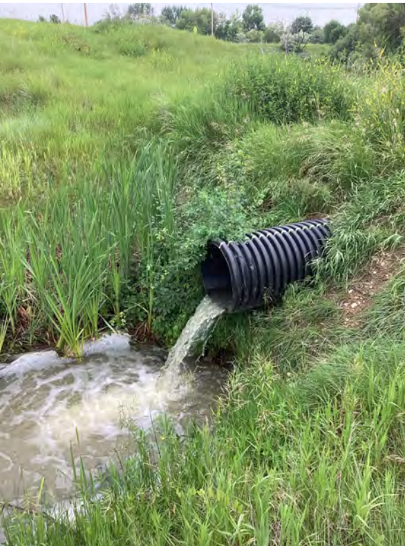
2.3 Holly No. 1 Reservoir - Reservoir Outlet (Looking Southwest)
