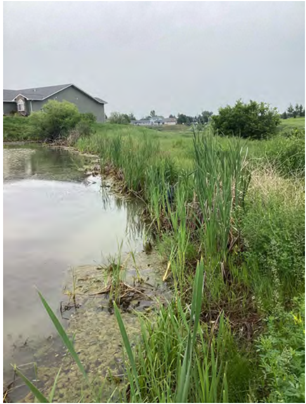
2.2 Holly No. 1 Reservoir - View of Dam (Looking Northeast)
