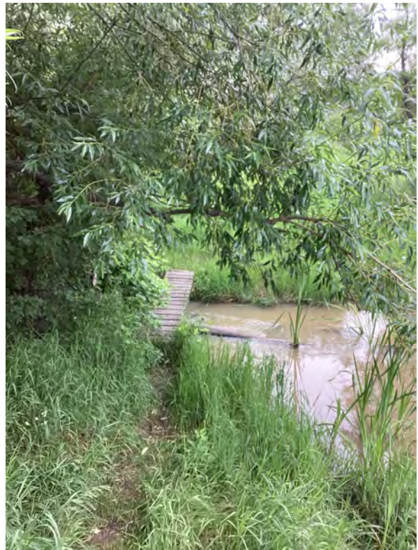
10.2 Unpermitted Reservoir - Emergency Spillway (Looking South)
