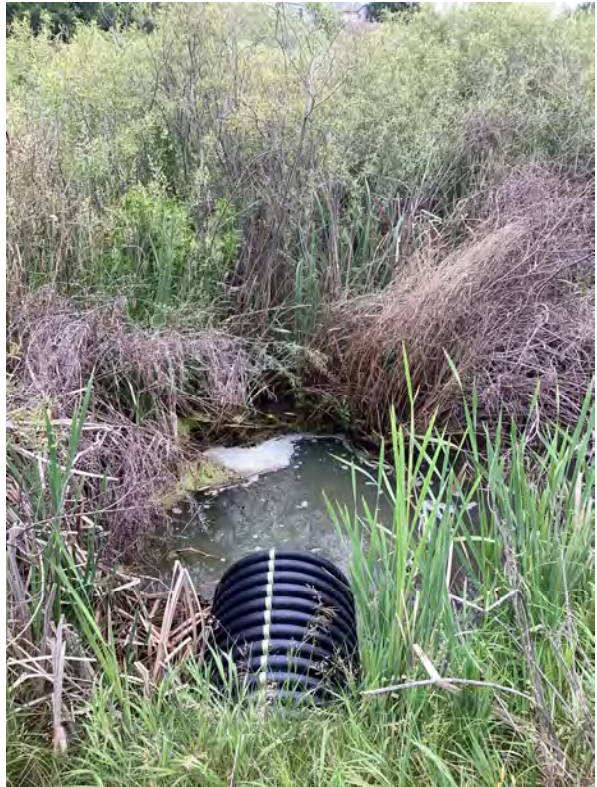
5.4 Holly Ponds No. 3 Reservoir - Outlet Culvert (Looking Northwest)
