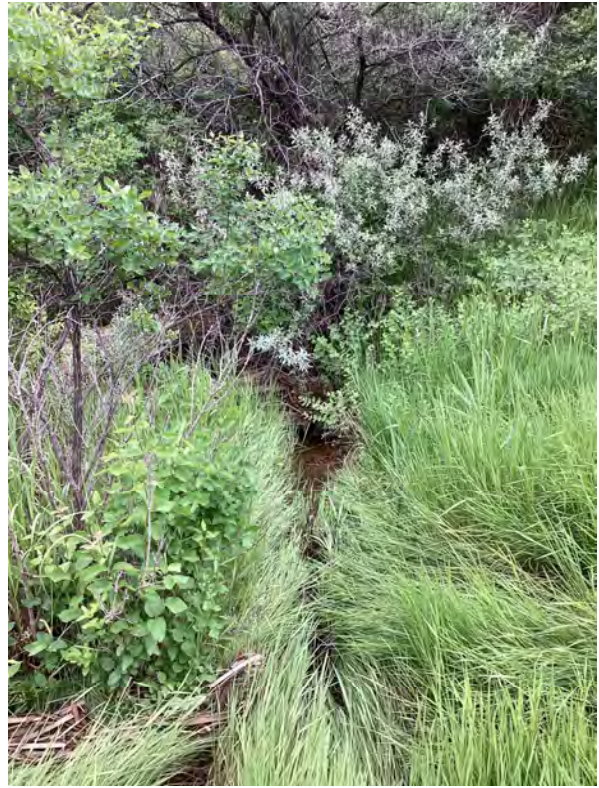
8.2 Holly No. 2 Reservoir - Emergency Spillway (Looking Southeast)
