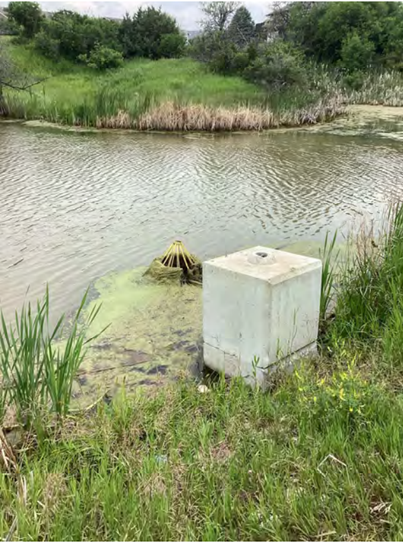
5.1 Holly Ponds No. 3 Reservoir - Outlet Structure (Looking West)
