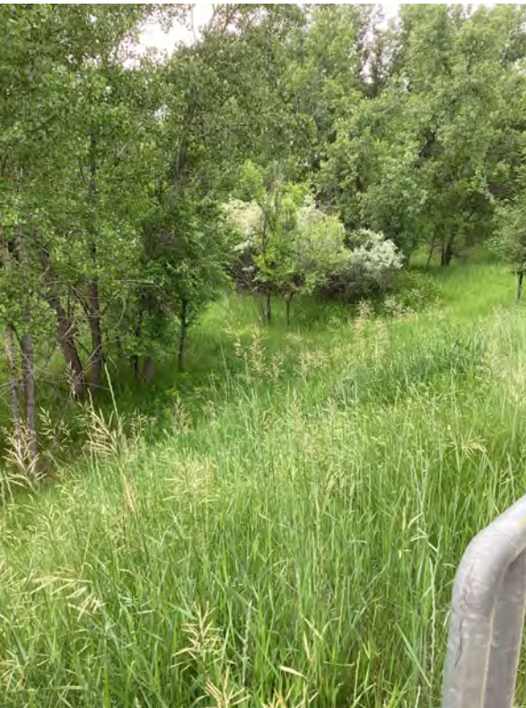
11.3 Mavrakis Pond - Emergency Spillway (Looking Southeast)
