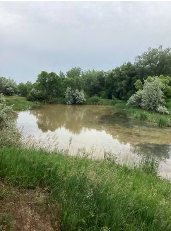
10.1 Unpermitted Reservoir - Reservoir View (Looking East)
