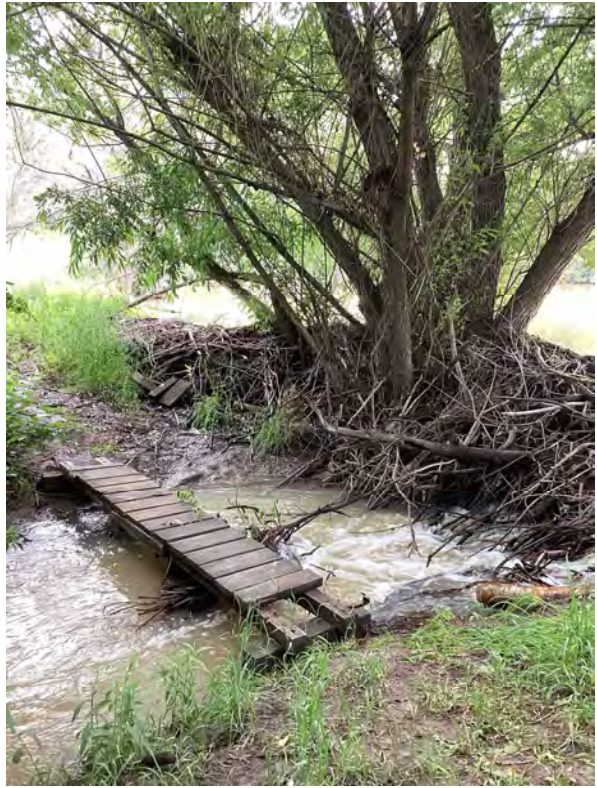
9.2 Hume No. 1 Reservoir - Emergency Spillway (Looking South)
