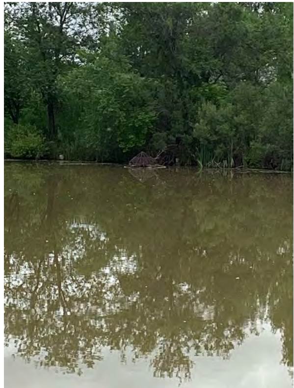
11.4 Mavrakis Pond - Trash Rack (Looking East)
