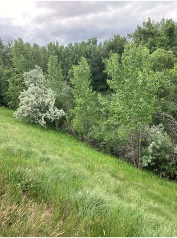
12.1 Hume No. 3 Reservoir - Reservoir View (Looking South)
