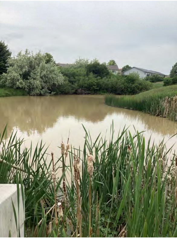
4.1 Holly Ponds No. 4 Reservoir - Reservoir Overview (Looking West)
