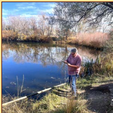
Water Treatment Superintendent Tom Manolis conducting a Dam Inspection
