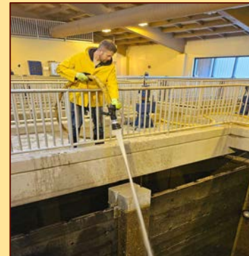
Will Litfin cleaning from the top of the basin at the Big Goose Water Treatment Plant
